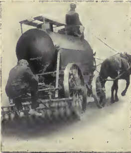
Monarch Pressure Oil Distributor. Furnished either in the horse-drawn type or for mounting on motor trucks.
